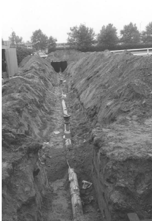
Fig. 6. (a) The test rig at UEA. (b) The UEA test rig under construction.
